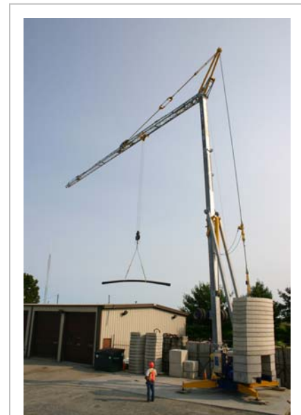
A Celtic self erecting crane 32.10
